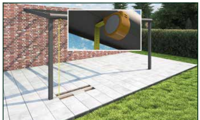
Gutter height from top of foundation column to flat underside of gutter
